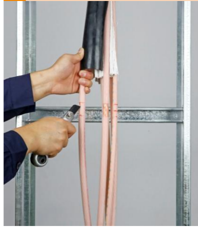
3 Stripping of main line insulation
