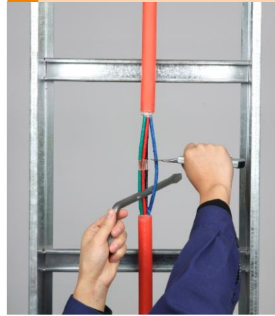
3 Stripping of main line insulation
