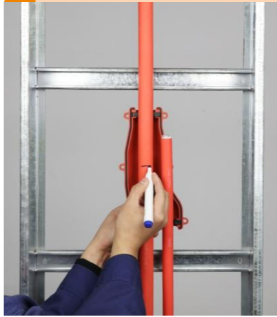
1 Determine the installation location
