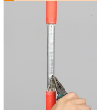
2 Strip away the outer sheath and metal layer
