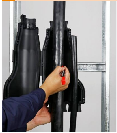
1 Determine installation location, strip outer sheath
