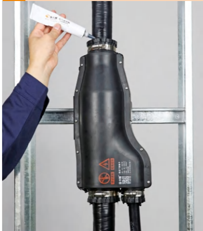
8 Lock and glue the cable outlet
