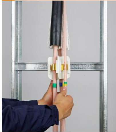
4 Installation of branch cable body
