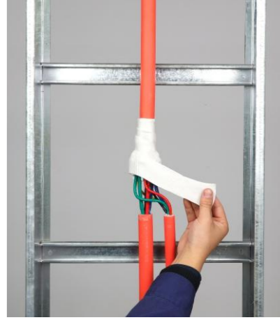
6 Overwrap mineral insulation refractory adhesive
