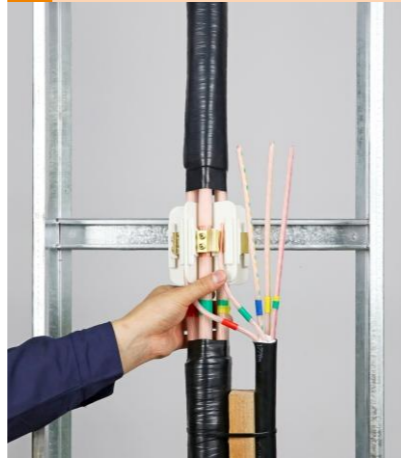
6 Installation of branch cables
