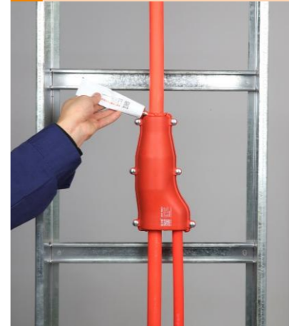
8 Lock and glue the cable outlet
